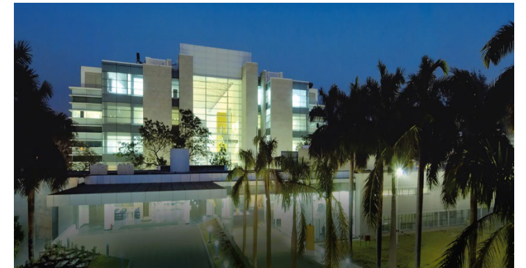
Implementation of Building Management And Safety Technology for a Life Sciences company
