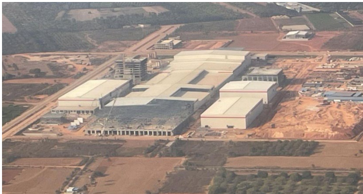
Integrated BMS and fire safety, security, and access control systems for a Giga factory
